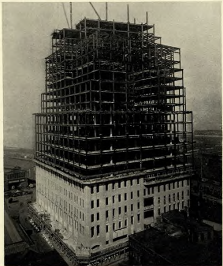
MASONRY ENCLOSING WALLS CLOSELY FOLLOWED THE STEEL SKELETON FRAME SKYWARD
