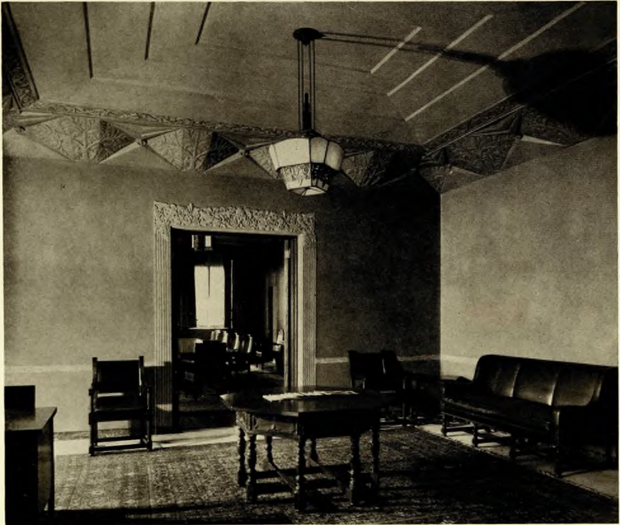
RECEPTION ROOM TO DIRECTORS' ROOM THE BARCLAY-VESEY TELEPHONE BUILDING, NEW YORK CITY MCKENZIE, VOORHEES & GMELIN, ARCHITECTS (See details on back)
