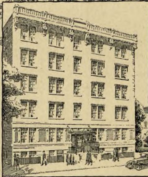
The Madison Apartments Elizabeth, N. J. C. Godfrey Poggie, Architect, built in 1926 by Berman Brothers for Mr. Welcome Bender
