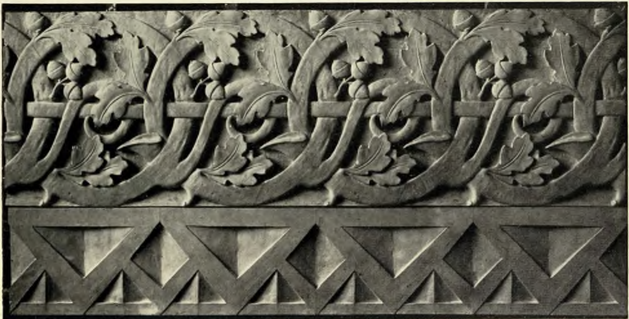
DETAIL OF EXTERIOR ORNAMENT AT 10TH FLOOR
