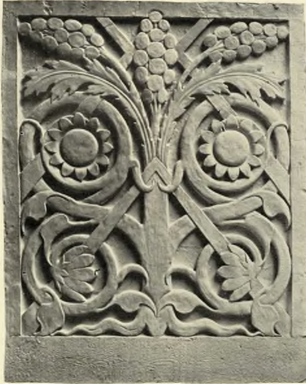
DETAIL OF EXTERIOR ORNAMENT AT 10TH FLOOR
