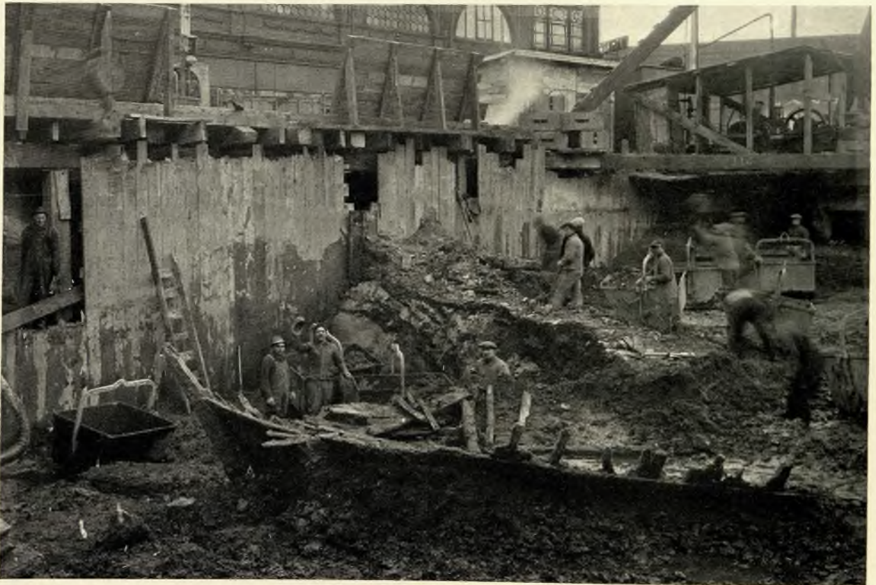
PORTION OF HULL OF AN OLD WHALING BOAT UNCOVERED IN EXCAVATING FOR THE FOUNDATIONS. AMONG OTHER RELICS OF THE PAST A WOODEN WATER MAIN DATING BACK TO THE EARLY DUTCH SETTLERS WAS UNEARTHED SIX FEET BELOW THE SURFACE ON VESEY STREET
