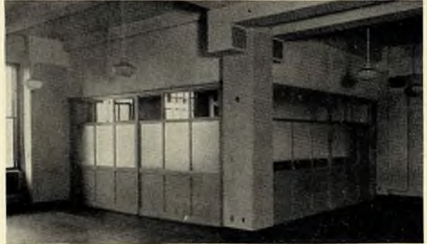
TYPICAL GENERAL CLERICAL SPACE. NOTE VENTILATING SUPPLY OUTLET NEAR CEILING. AIR IS EXHAUSTED THROUGH DUCTS CUT OFF ONE FOOT ABOVE THE FLOOR. ONE OF THESE DUCTS CAN BE SEEN AT THE EXTREME RIGHT
