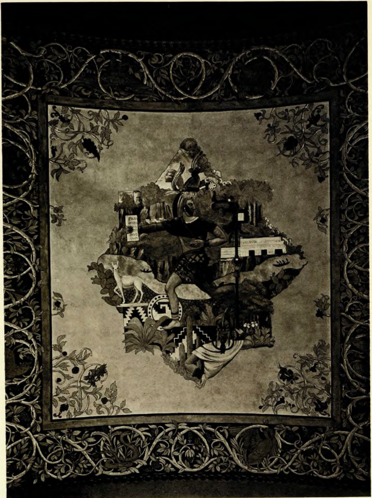
DETAIL OF ONE OF A SERIES OF DECORATIVE CEILING PANELS IN THE MAIN CORRIDOR. BY MACK, JENNEY & TYLER
