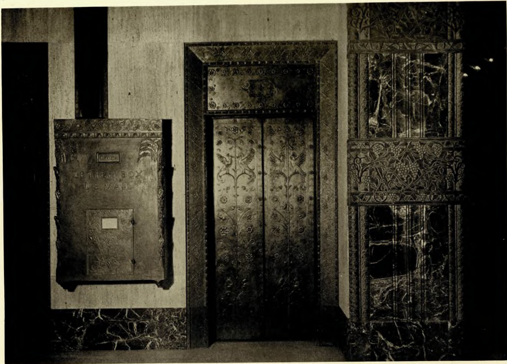
DETAIL OF ELEVATOR DOORS AND LETTER BOX IN MAIN CORRIDOR THE BARCLAY-VESEY TELEPHONE BUILDING, NEW YORK CITY MCKENZIE, VORHEES & GMELIN, ARCHITECTS
