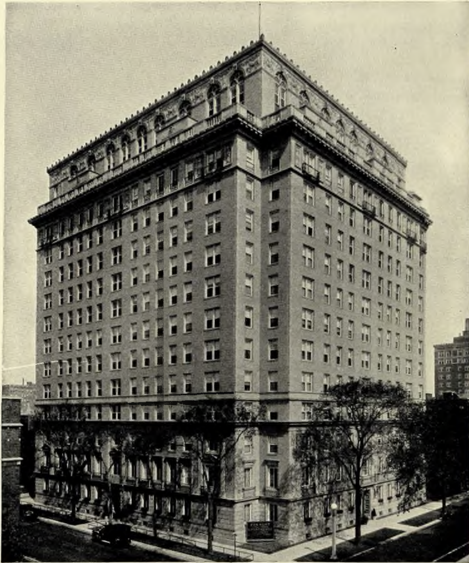
The Barry Apartments, Chicago, Ill., Robert S. DeGolyer & Co., Architects
