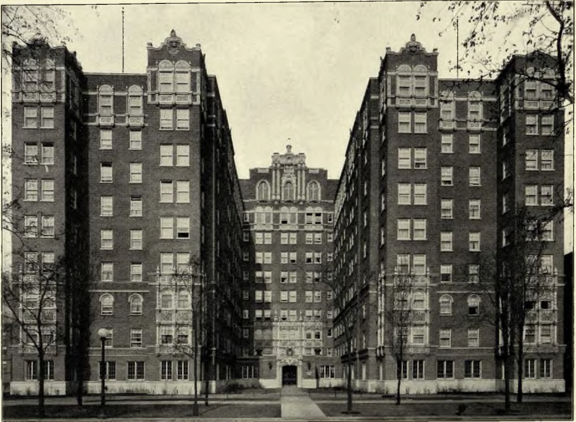
Country Club Apartments, South Shore Drive, Chicago. Hall, Lawrence, Rippel & Ratcliffe, Architects.
