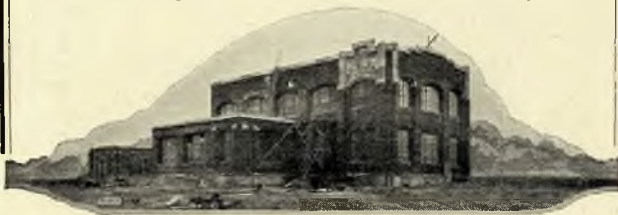
NEW PUMPING HOUSE Municipal Water Plant Kansas City, Mo.
