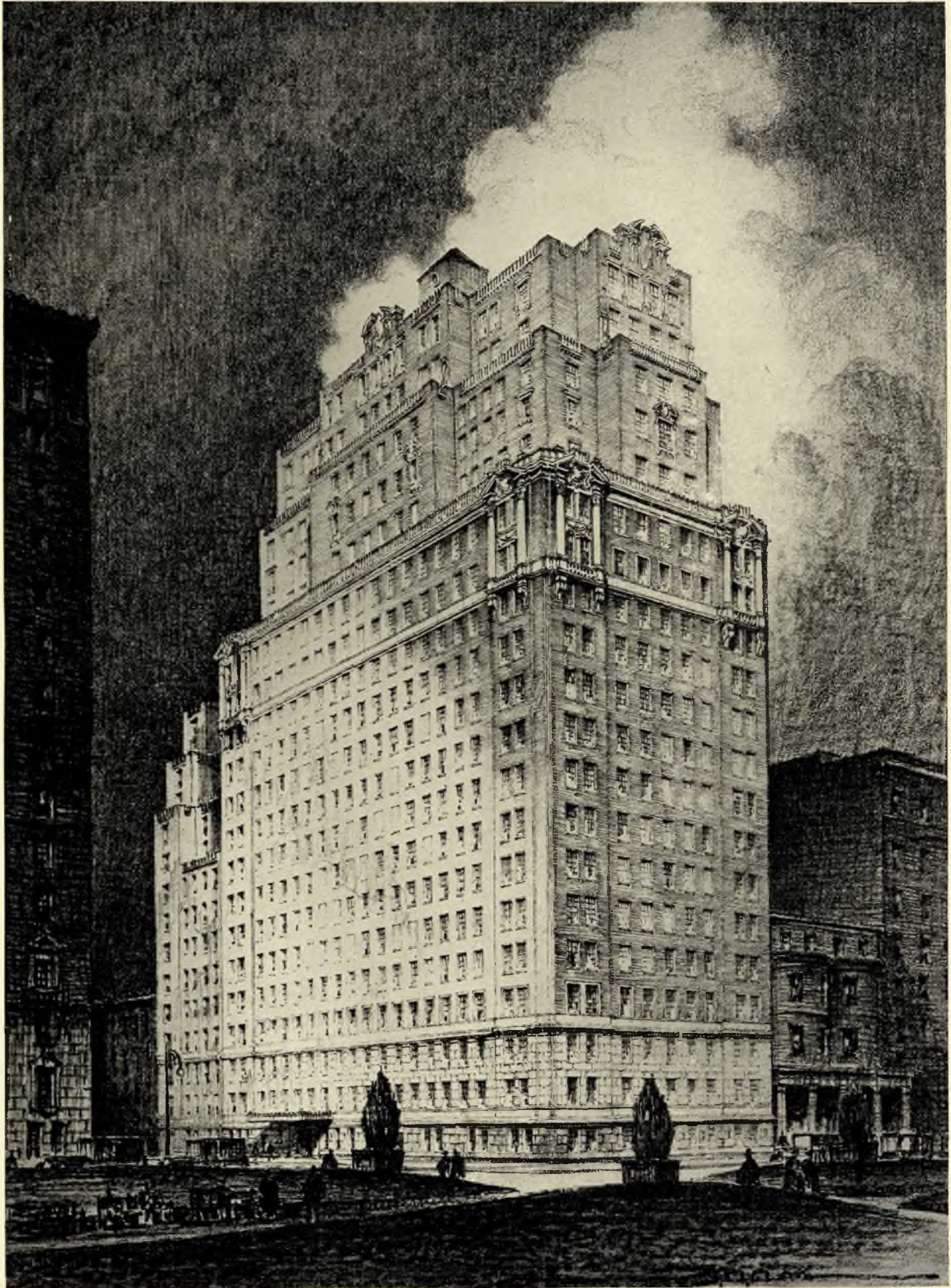
THE DRAKE, AN APARTMENT HOTEL AT 440 PARK AVENUE, NEW YORK
