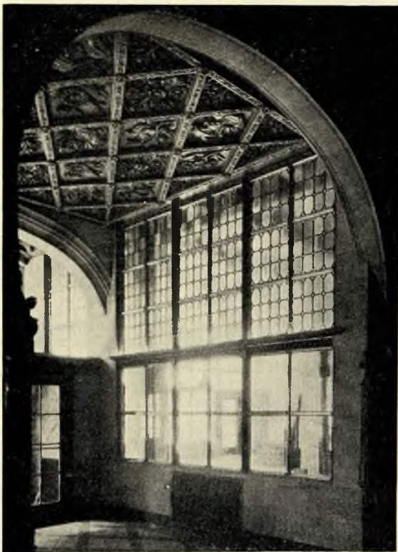
Interior—Imitation stone work, also executed by G. E. Walter Duretta Ceiling—Cellini Building, 48 West 48th St., New York City James C. Green, Architect
