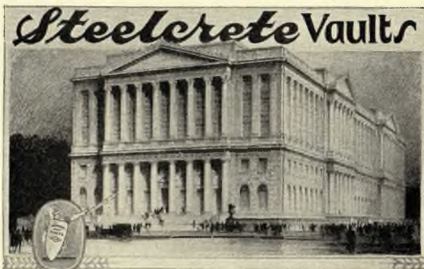
The magnificent new home of the Mutual Benefit Insurance Company at Newark, N. J. Its modern vault is protected by 345 tons of Steelcrete Armor Mat. J. H. & W. C. Ely, Newark, Architects; Starrett Bros. Inc., New York, Contractors.
