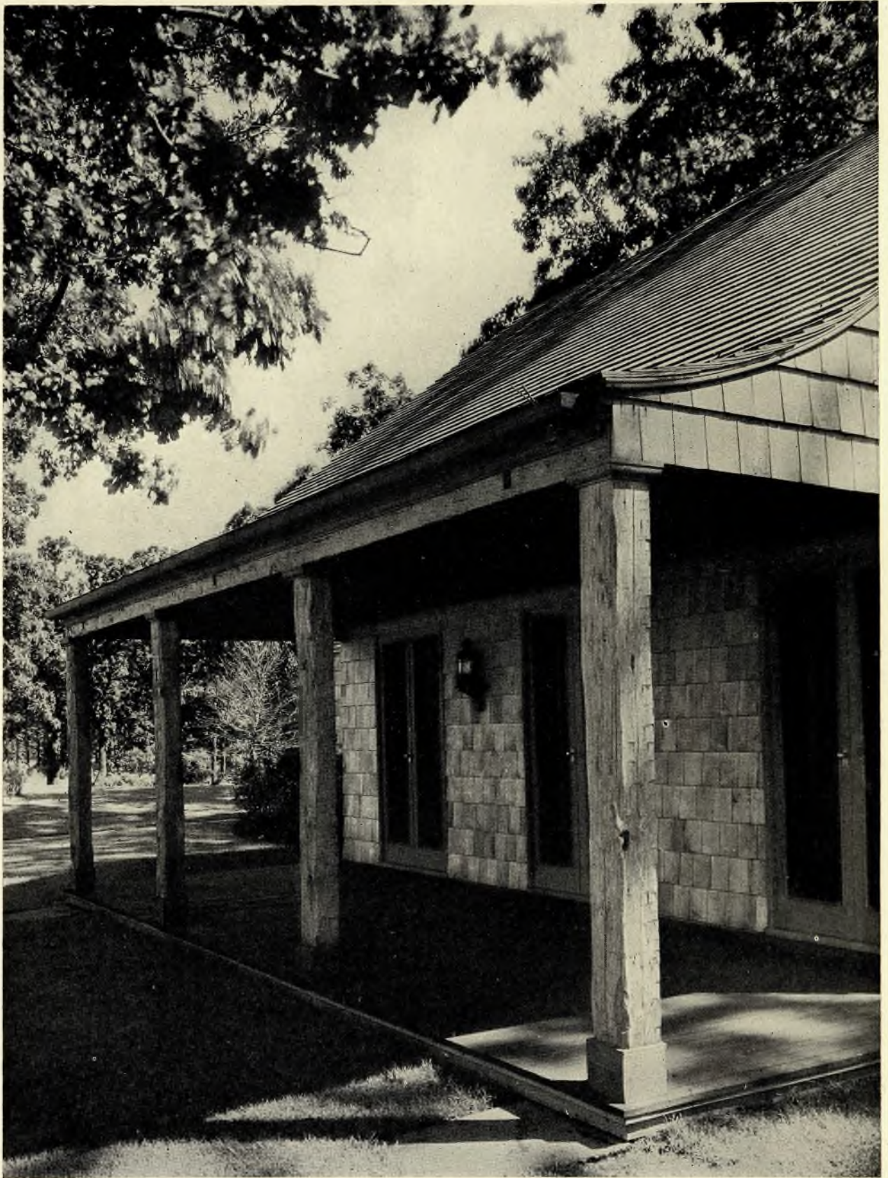
BATH HOUSE ON ESTATE OF MARSHALL FIELD, LONG ISLAND, N. Y.
