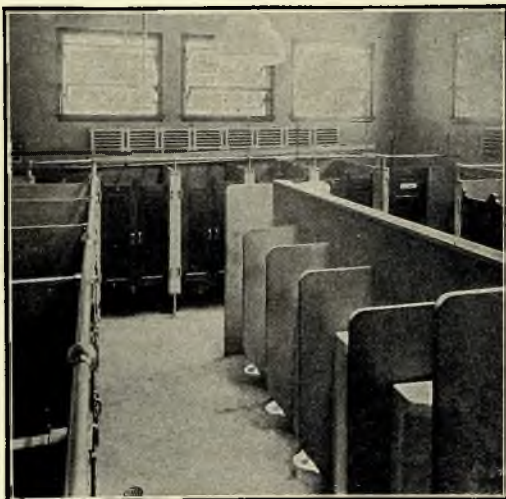
Sanitary work in Alberene Stone in the Louisiana Avenue Comfort Station, Baltimore, Maryland
