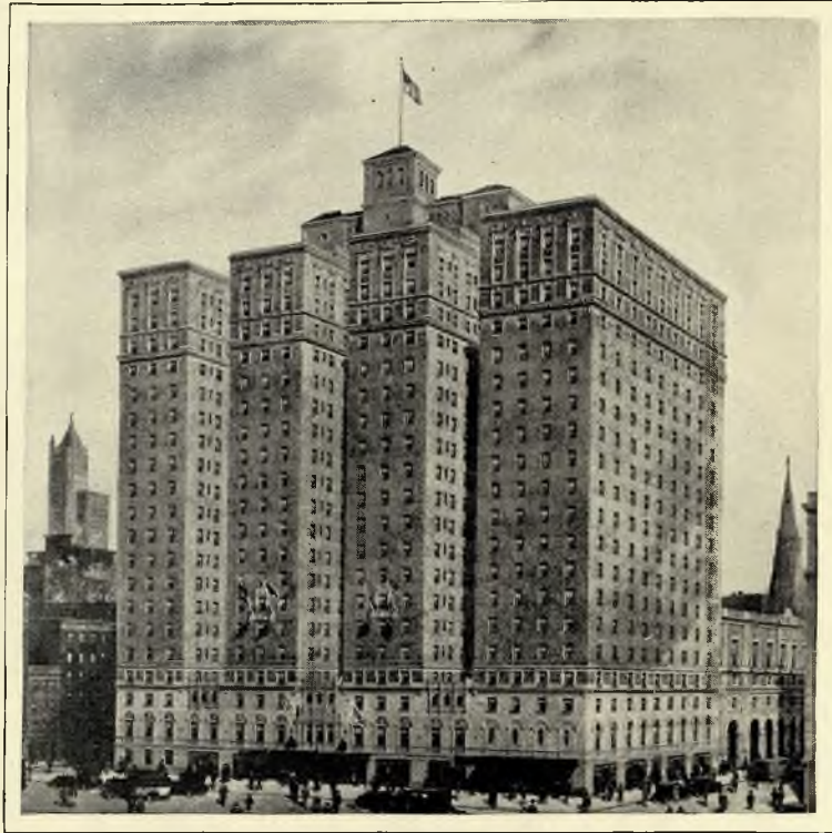
HOTEL MANGER, New York City: H. Craig Severance, New York, Architect; E. Smolka Plumbing Supply Co., New York, Jobbers; Jarcho Brothers, New York, Plumbers
