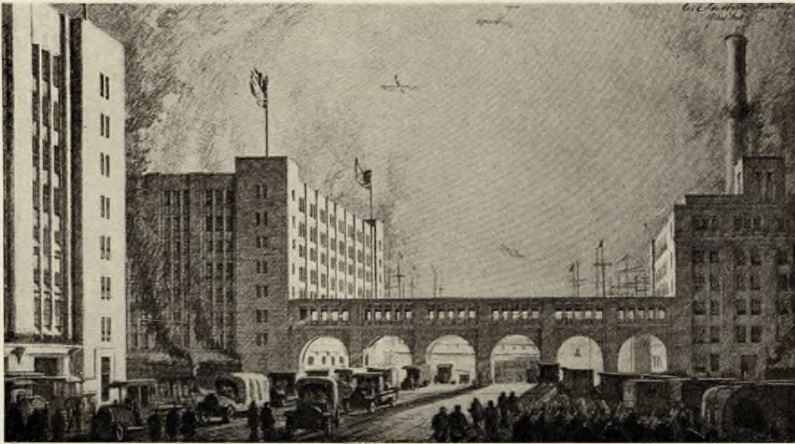
LOOKING TOWARDS THE WATER FRONT AND PIER 4. WAREHOUSE A ADMINISTRATION BUILDING AND CONNECTING BRIDGE
