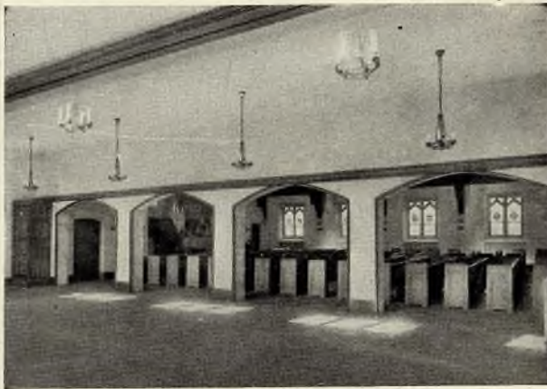
ALL PARTITIONS FOLDING AT THE END OF ROOM Folding Partitions as installed in the Church of the Evangel, Brooklyn, N. Y.
