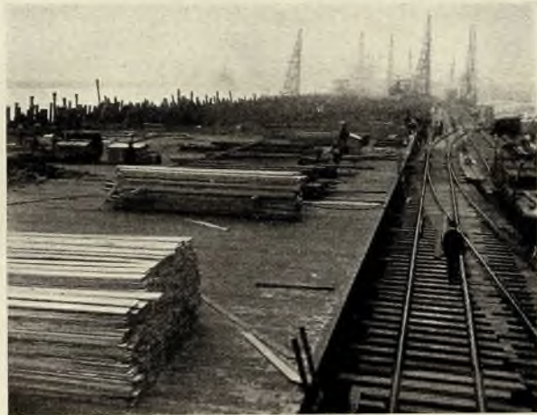
No. 2. FEBRUARY 19, 1919. DECKING LAID OVER COMPLETED PILES.
