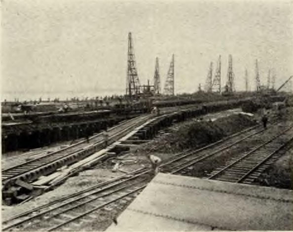
No. 1. JANUARY 22, 1919. PILE DRIVING IN PROGRESS.
