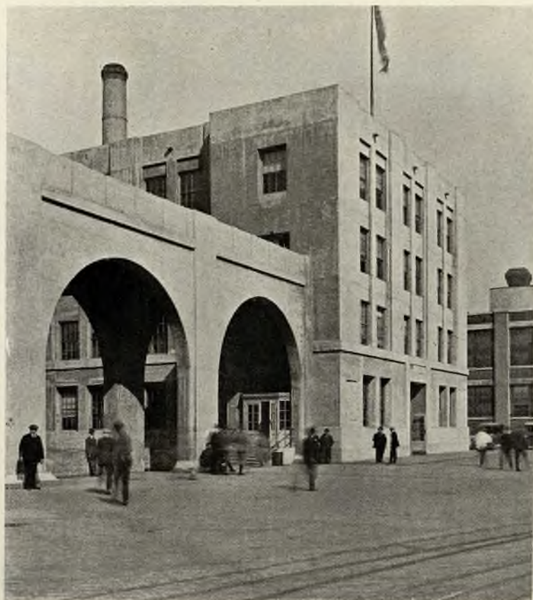
A WAREHOUSE AND CONNECTING BRIDGE
