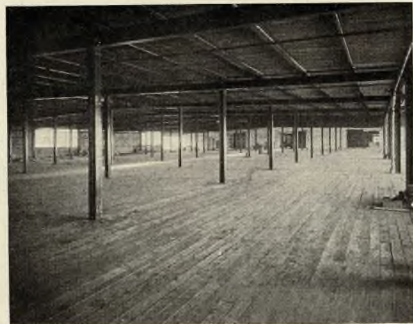
No. 6. INTERIOR VIEW OF COMPLETED WHARFHOUSE.
