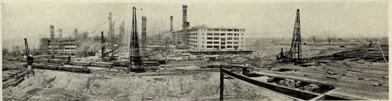
VIEW OF WAREHOUSES SIX WEEKS LATER, SHOWING RAPID CONSTRUCTION ATTAINED.
