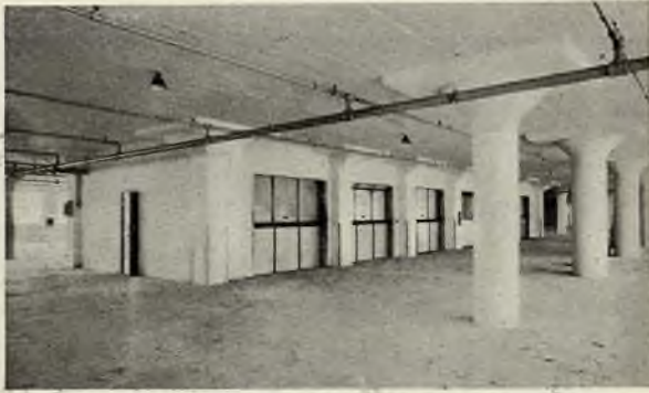
INTERIOR VIEW OF WAREHOUSE SHOWING ONE OF THE ELEVATOR BATTERIES.
