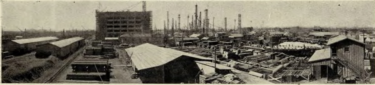
WAREHOUSES 1, 2 AND 3 AS THEY APPEARED JANUARY 15, 1919.
