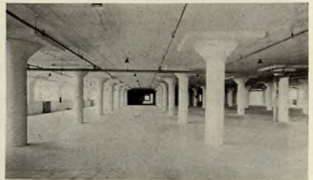
TYPICAL INTERIOR VIEW OF WAREHOUSE. INTERIOR CONSTRUCTION IDENTICAL FOR ALL WAREHOUSES.
