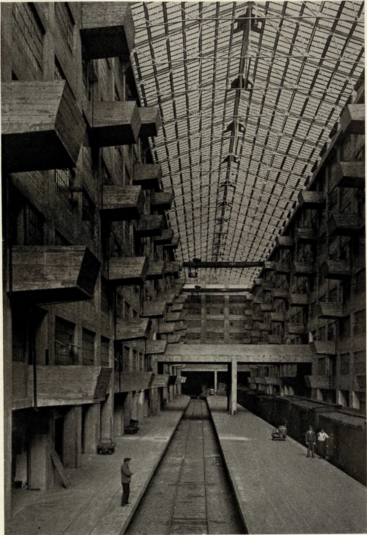
Court in Building B, showing arrangement of cantilever balconies served by travelling cranes, handling supplies direct from rail to warehouse. PLATE 184 UNITED STATES ARMY SUPPLY BASE, BROOKLYN, N. Y. CASS GILBERT, ARCHITECT
