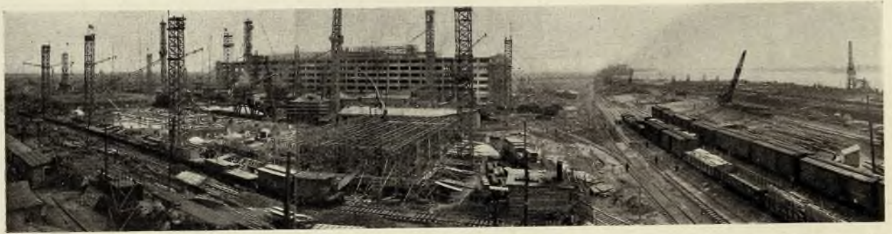
GENERAL VIEW OF SITE, SHOWING CONDITION AS IT APPEARED FEBRUARY 12, 1919
