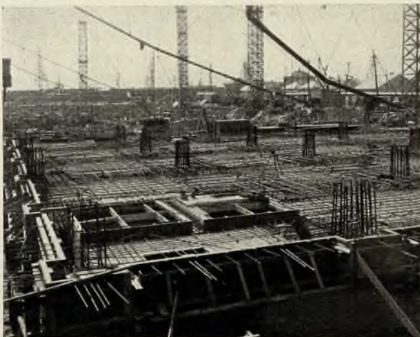
WHARFHOUSE NO. 3 AS IT APPEARED JANUARY 15, 1919.
