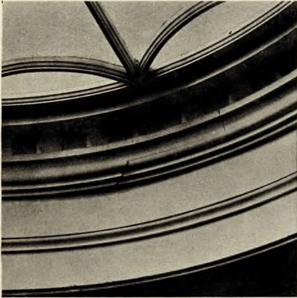
TYPICAL EXAMPLE OF TANGENTIAL AND LONGITUDINAL SHRINKAGE IN MOULDINGS CUT TO A RADIUS
