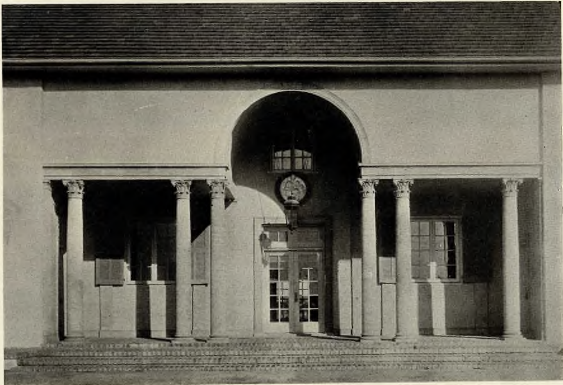
DETAIL OF MAIN ENTRANCE
