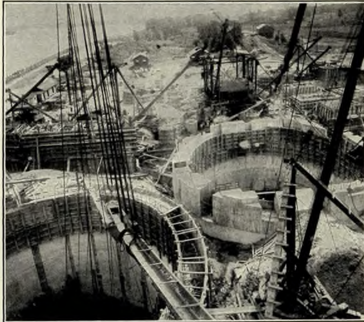
NEW PLANT KANSAS CITY LIGHT AND POWER CO.
