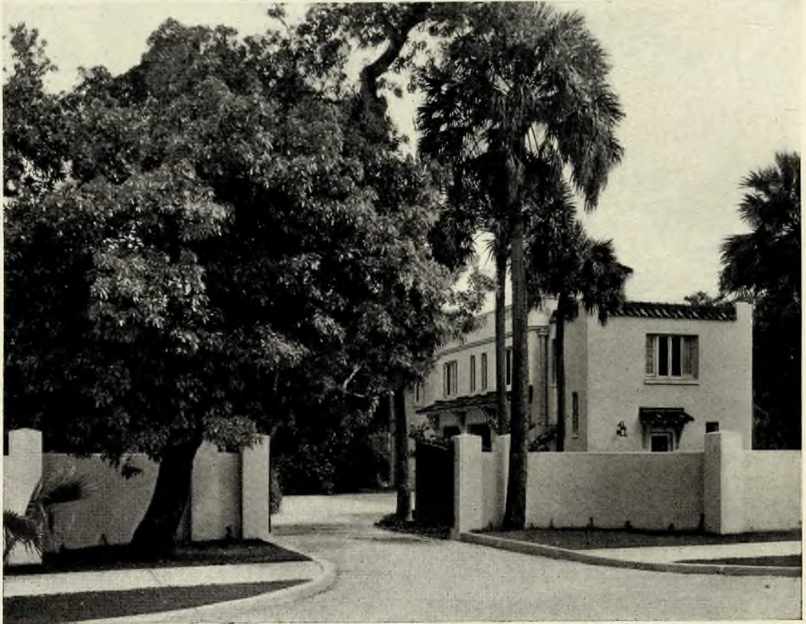
MAIN ENTRANCE AND GARAGE
