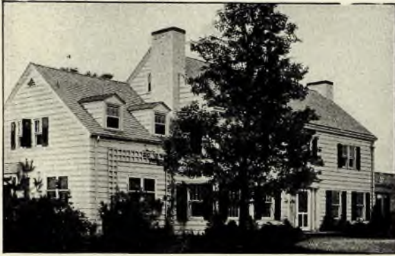
Walls finished with Cabot's Old Virginia White Roof Stained with Cabot's Creosote Stains. J. W. O'Connor, Architect, N. Y.
