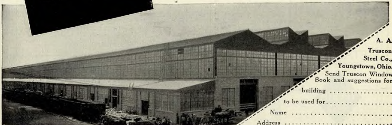
Erection building of Ford Eagle plant, 1700 feet long, 250 feet wide. Four acres of Truscon Steel Windows. Albert Kahn, Architect.
