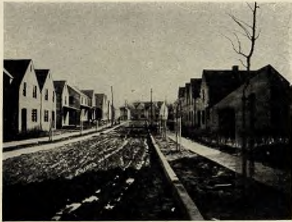
STREET NO. 3, LOOKING NORTH
