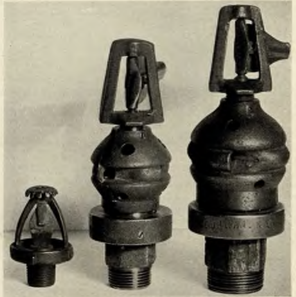
Automatic Sprinkler Heads
