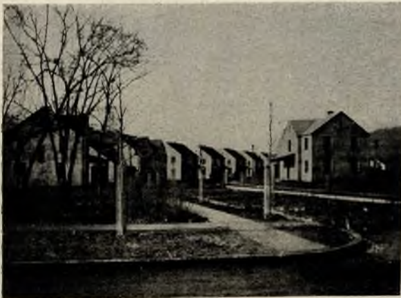
STREET NO. 2, LOOKING WEST
