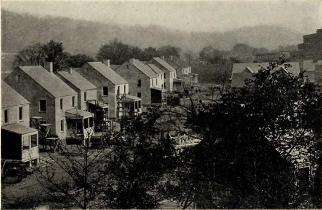
REAR OF HOUSES ON STREET NO. 5
