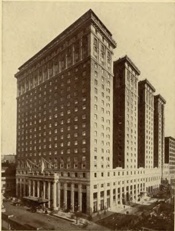
PENNSYLVANIA HOTEL, NEW YORK Architects: McKim, Mead & White Equipped with Otis Elevators
