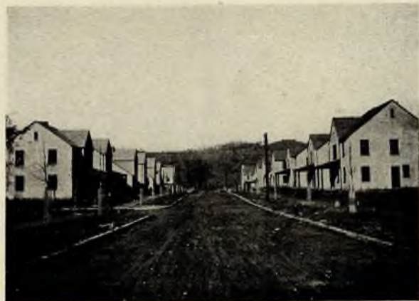
STREET NO. 1, LOOKING NORTH
