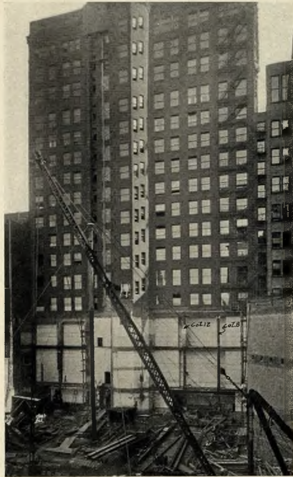
NEW GUARDIAN BUILDING, CLEVELAND View from Vincent Street
