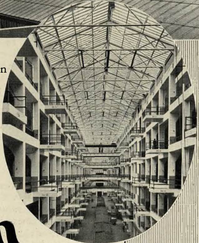
Ford Motor Co., Detroit, Mich. Radiator and Upholstery Depts. 73,000 sq. ft. Lupton Rolled Steel Skylight used.
