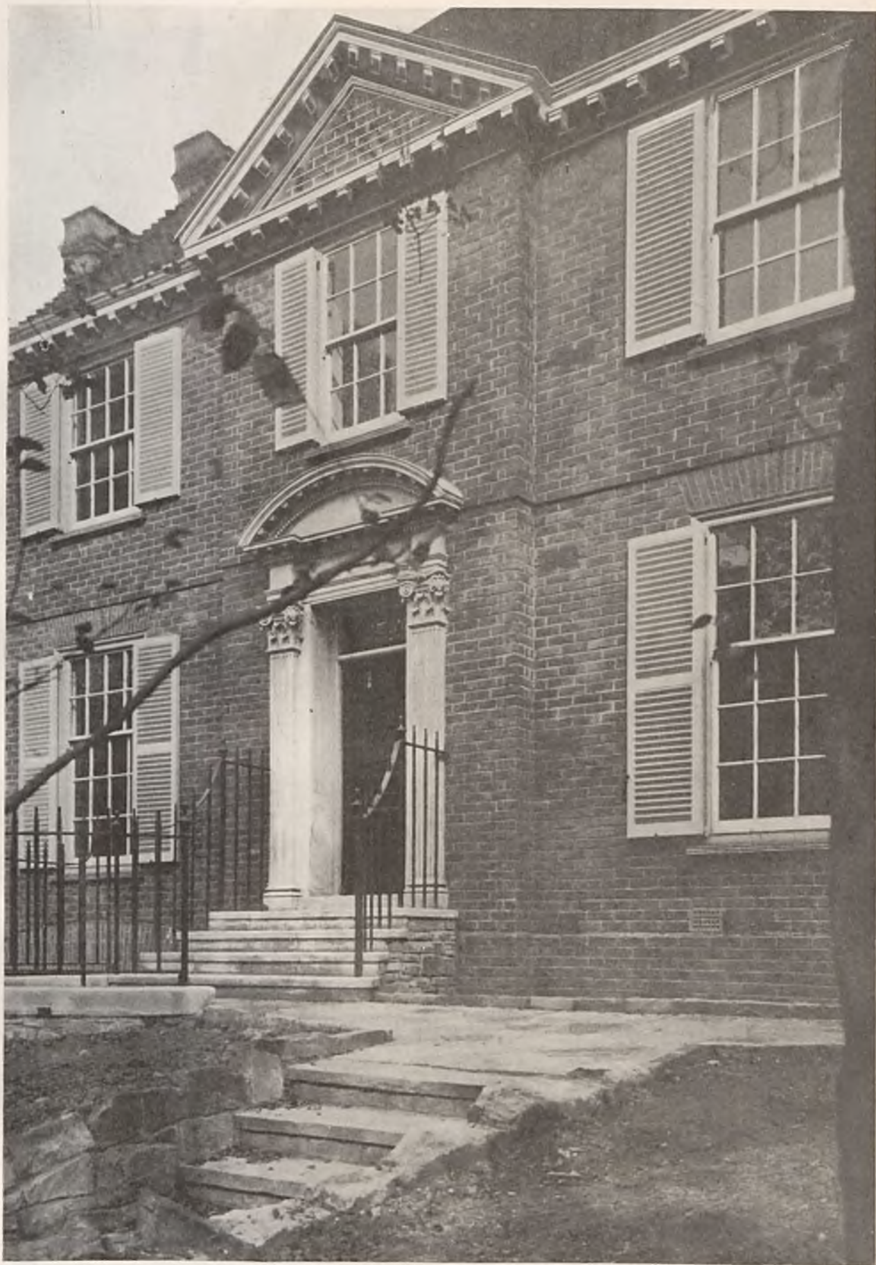
House in Finchley Road, N.W.: Detail of Entrance Front.
