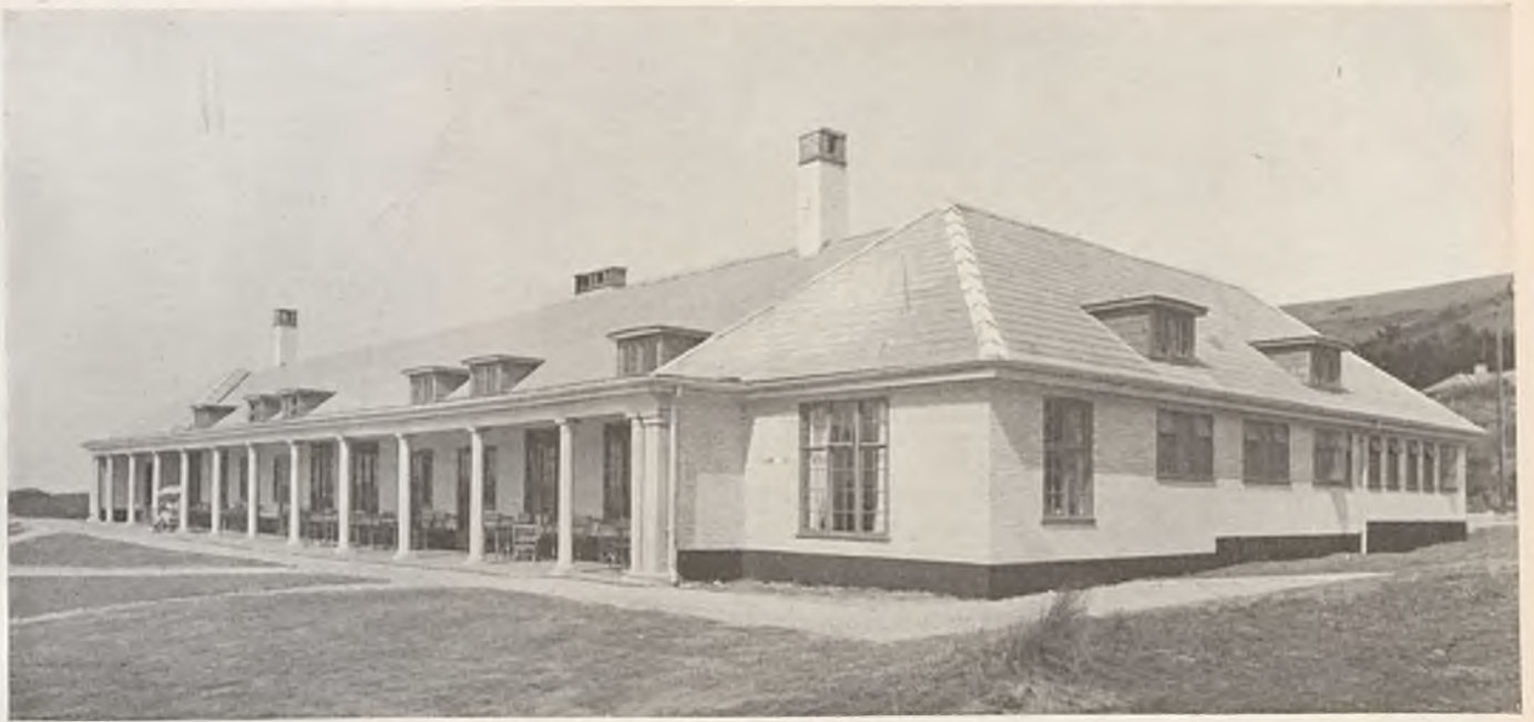
GENERAL VIEW OF EXTERIOR.
