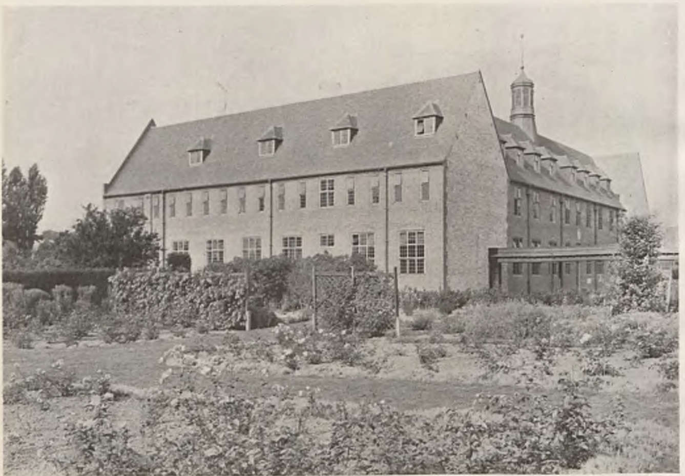
GENERAL VIEW FROM SOUTH-WEST.
