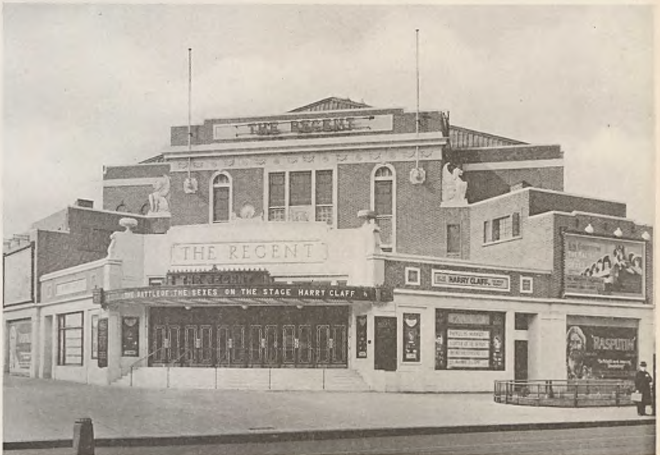
GENERAL VIEW OF EXTERIOR.
