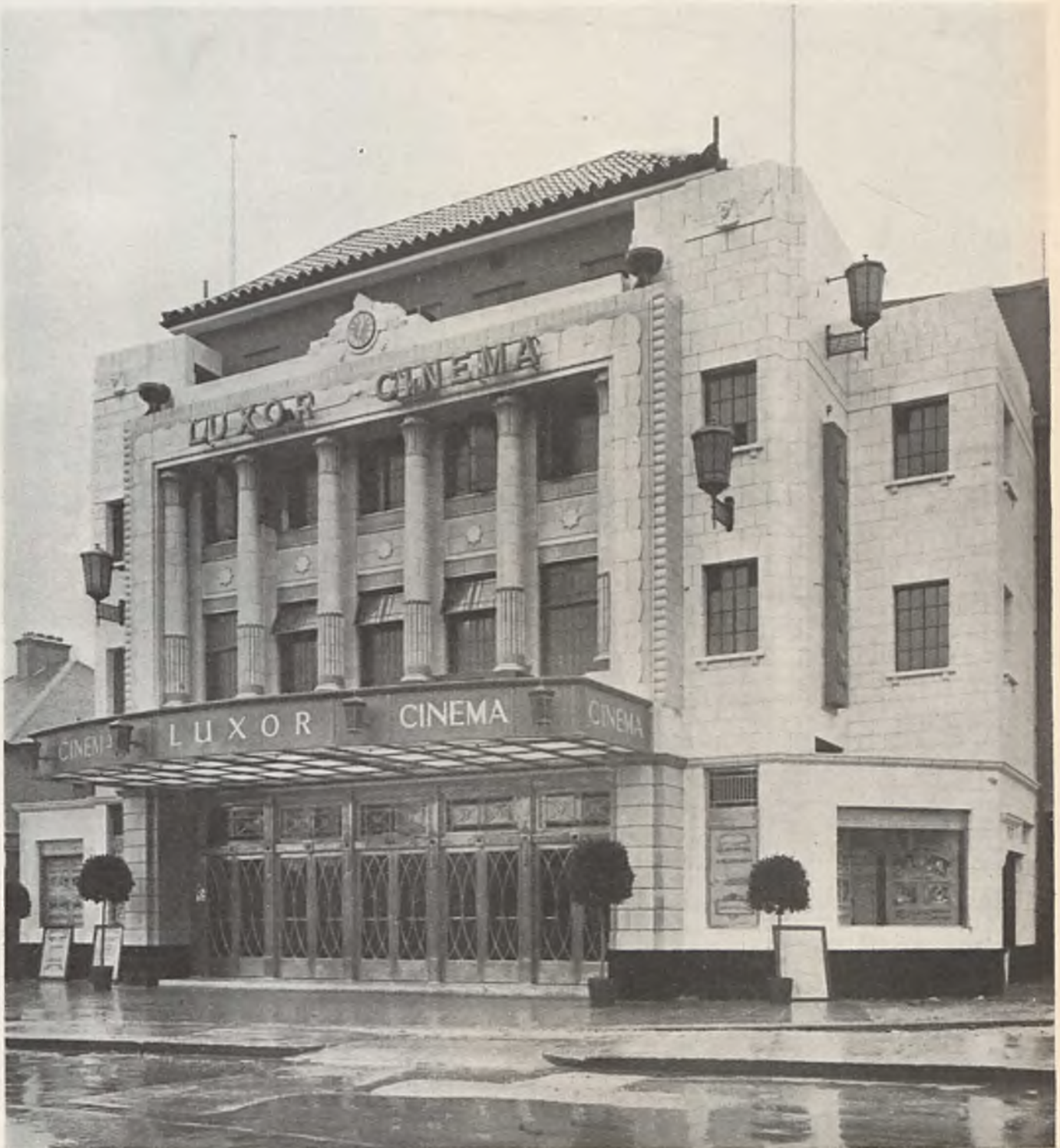
The "Luxor" Cinema, Twickenham: General View of Exterior.
