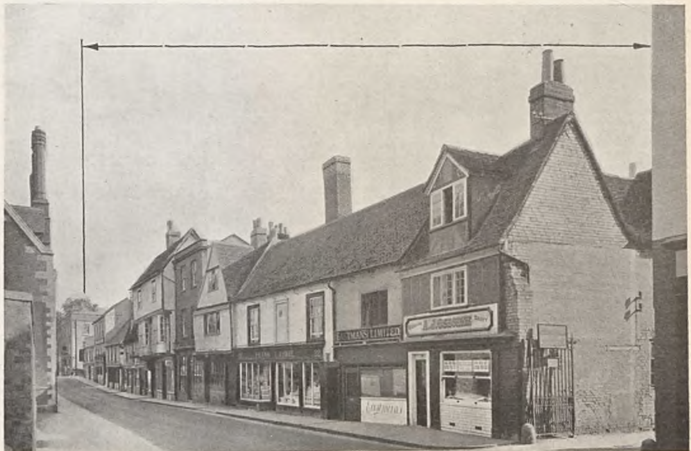
Old Houses in Magdalene Street, Cambridge. Property between vertical lines is to be pulled down.
