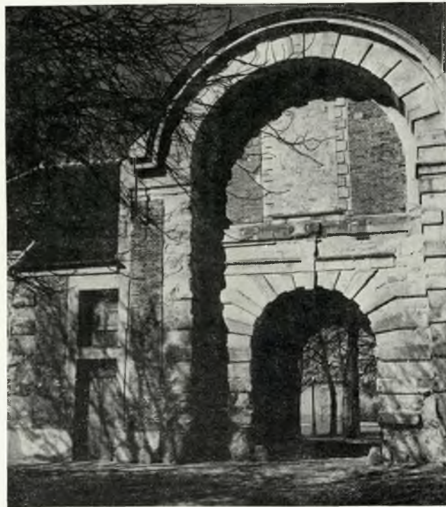
FIG. 17.—Château of Montceaux-en-Brie, Central entrance, south range of forecourt.
