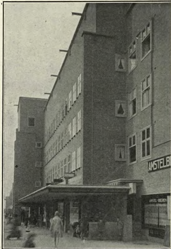
Fig. 6.—IN THE NEW SUBURB OF AMSTERDAM. A DETAIL OF THE MARQUISE: THE CLERESTORY LIGHTS TO THE SHOPS ARE VISIBLE ABOVE THE SHELTER.
