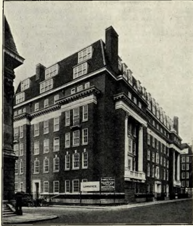
NEW FLATS, PARK STREET, W. Messrs. WIMPERIS, SIMPSON & GUTHRIE, F.F.R.I.B.A., Architects.
