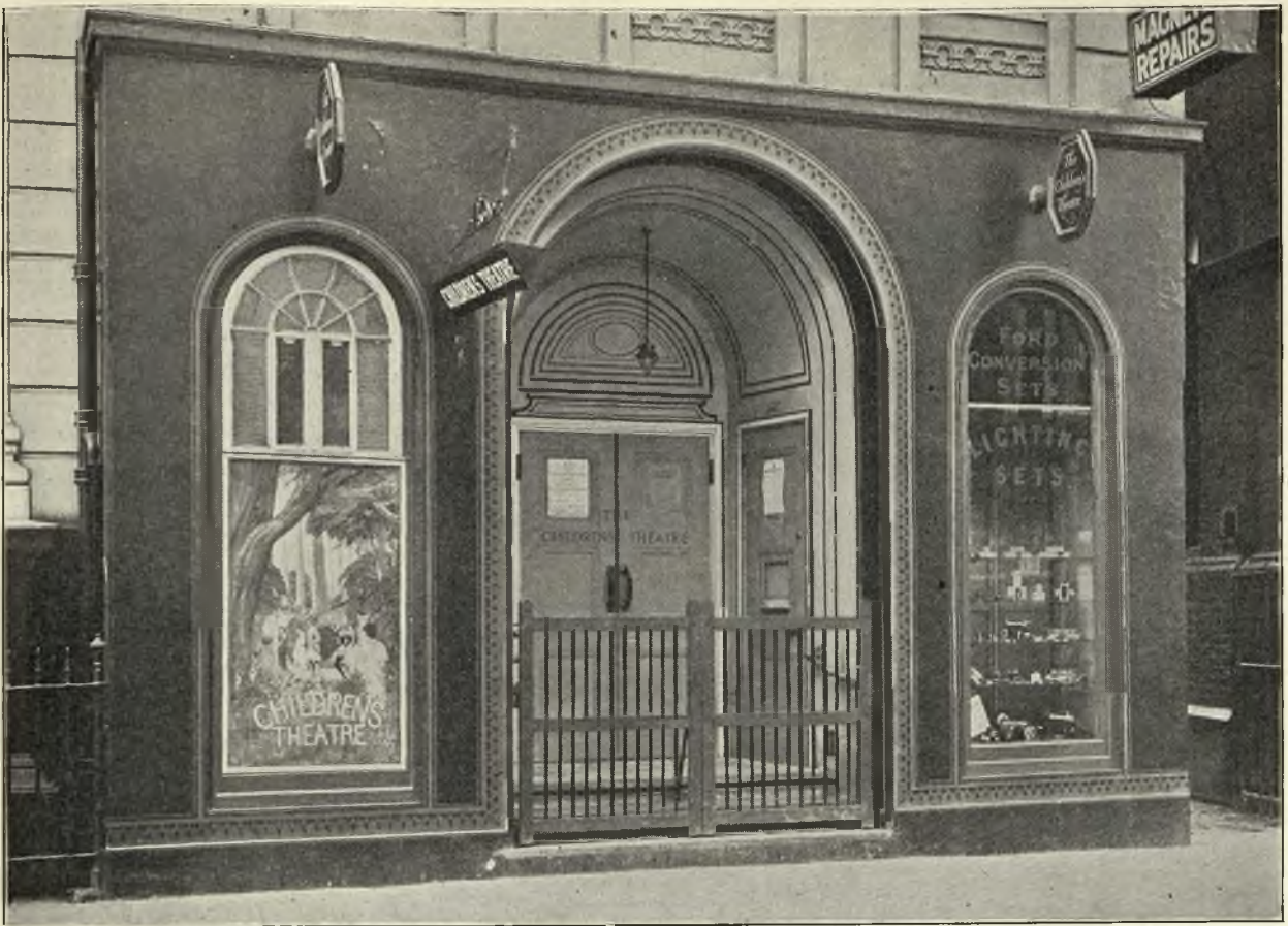
THE CHILDREN'S THEATRE, ENDELL STREET, W.C.2. W. BRAXTON SINCLAIR, F.R.I.B.A., Architect.
