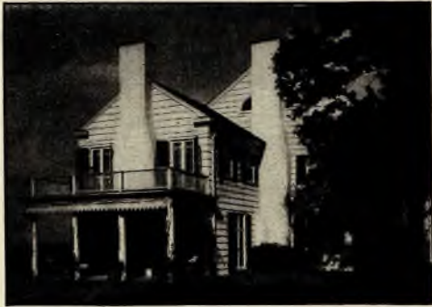
Brick Chimneys and Wall Shingles finished with Cabot's Old Virginia White John Russell Pope, Architect, New York
