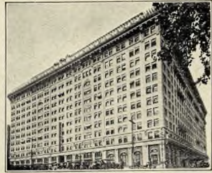
The Hotel Du Pont, Wilmington, Del., Speakman Company, Wilmington, Del., Jobbers; Alexander Bryant & Co., New York City, Plumbers
